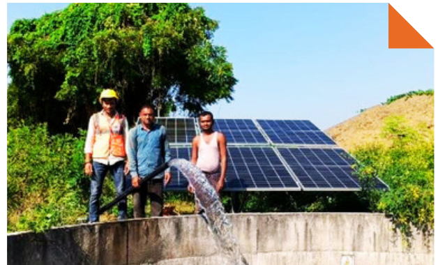
MSEDCL 1291 nos Solar Water Pump
