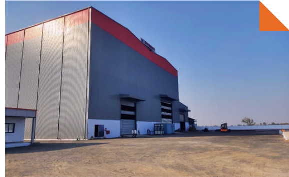
Thermotech Systems Limited (149.60 kWp)
