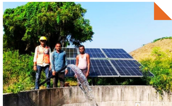
MSEDCL (1291 Nos. Solar Water Pump)
